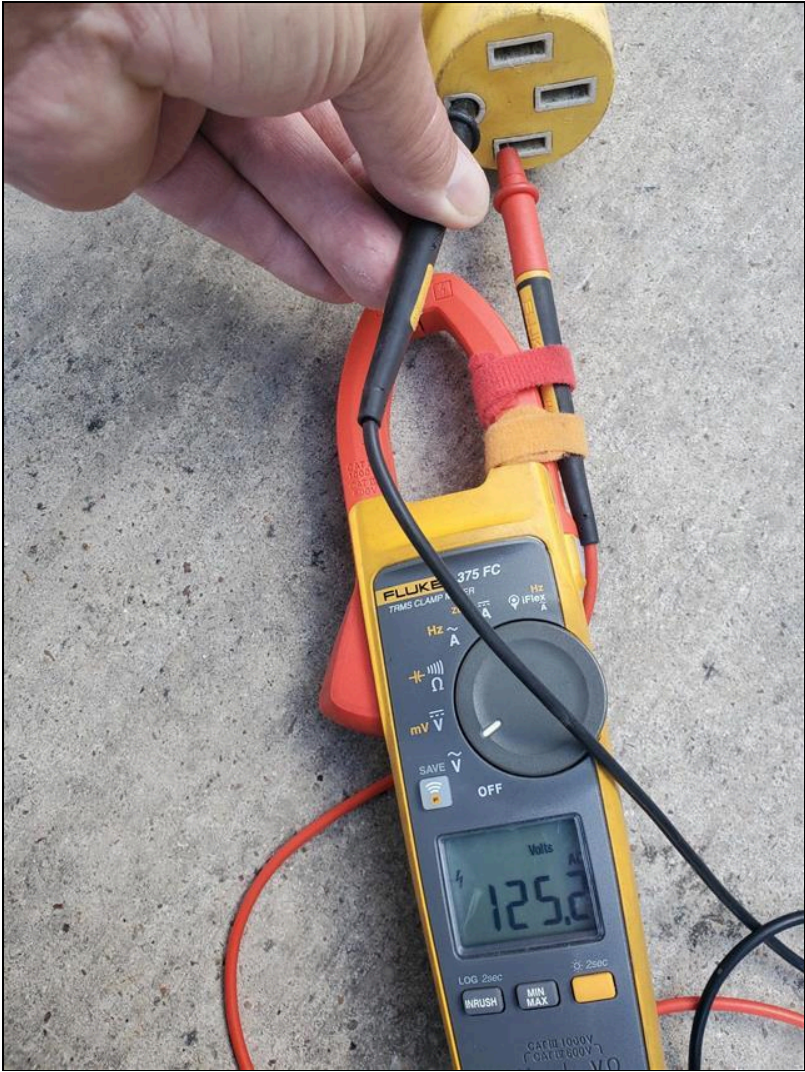
Power at Pedestal Verified Before Testing Unit
